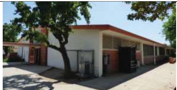
North & East Elevations of Building 5, View South West
