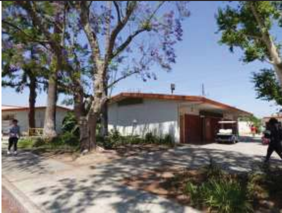
Building 13, West and South Elevations, View East
