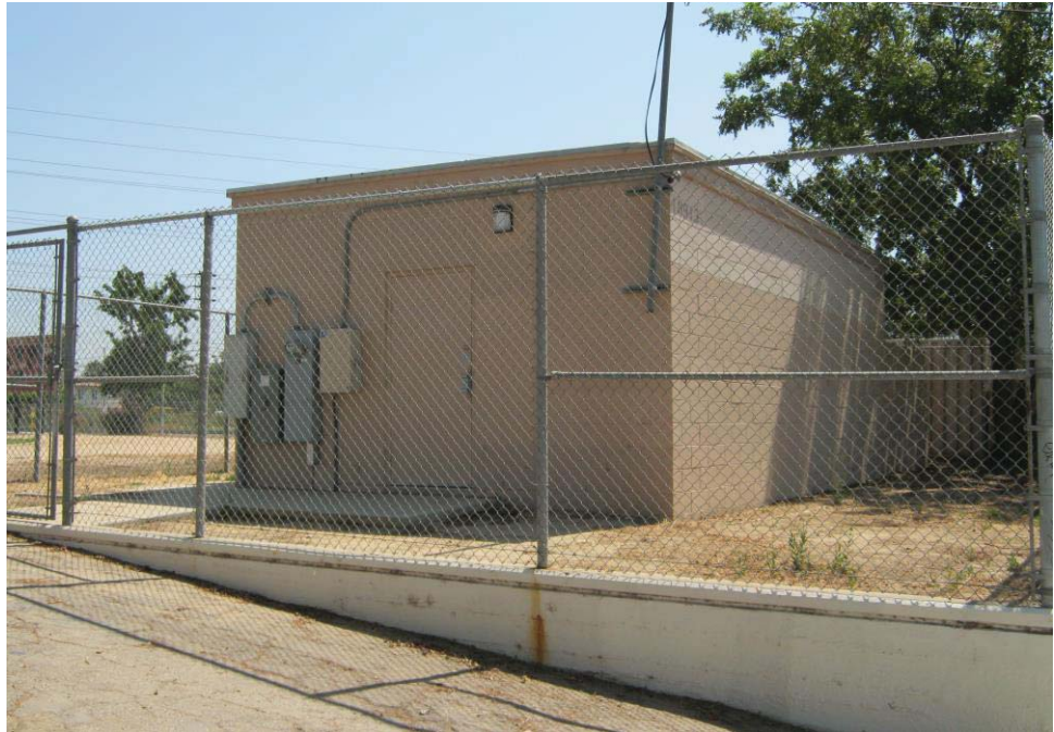
Photograph 5: View of former fiber optic hub building in the southeast portion of the site.
