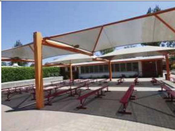
Building 17, North Elevation, View South
