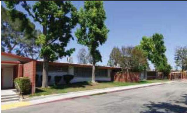
Classroom Building 3, South Elevation, View Northeast
