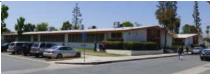
Classroom Buildings 7 to 10, View Northwest
