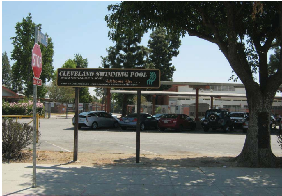
Photograph 3: Looking east at the Cleveland Swimming Pool.
