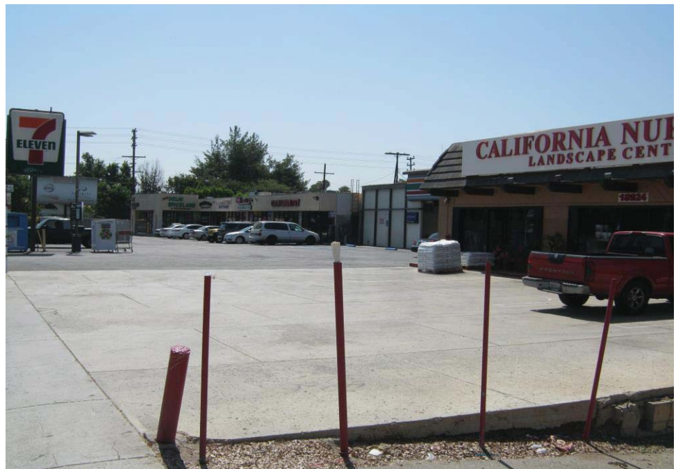
Photograph 22: Looking east away from the Aliso Canyon Wash at a strip mall (former Thrifty #0069 gasoline service station).
