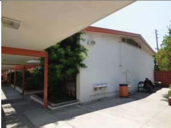
Library Building 2, North Elevation, View South
