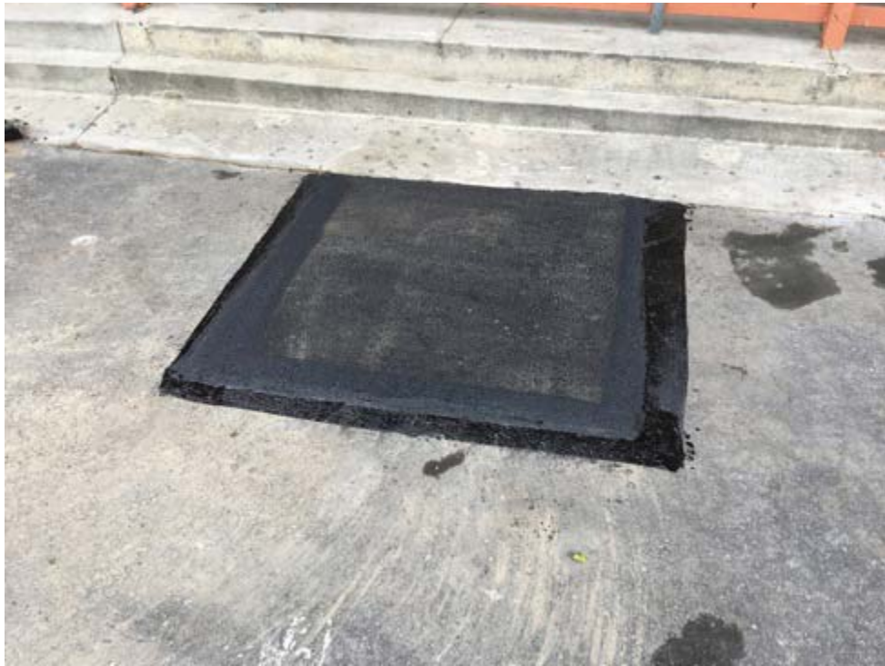
Photograph 8 – Vapor probe SV2 excavation after backfilling and paving.
