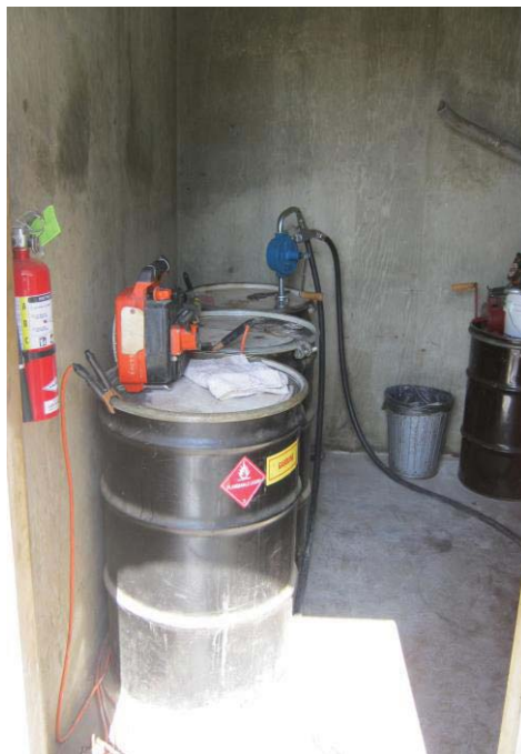
Photograph 8: View of 55-gallon drums of diesel and gasoline in the storage room of the custodian building.
