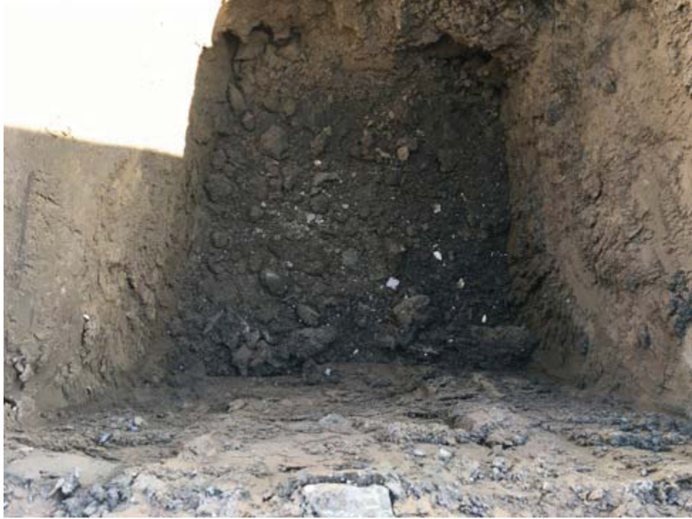
Photograph 7 – Vapor probe SV2 after excavation, second view.
