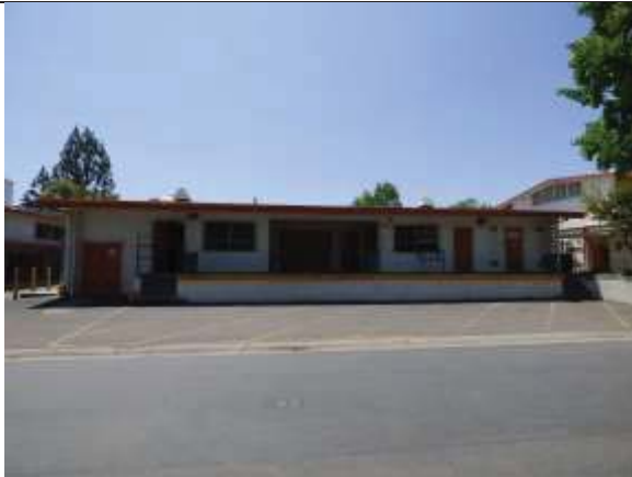
Building 18, East Elevation, View West
