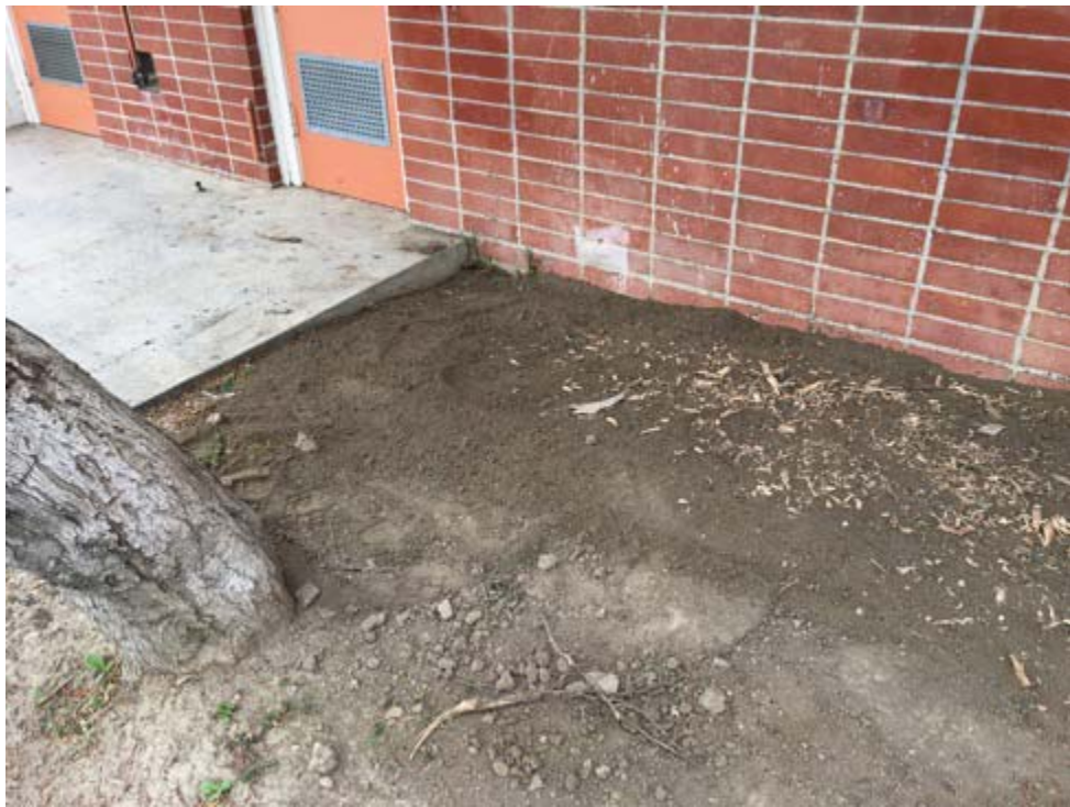
Photograph 4 – Boring B37 after backfilling.
