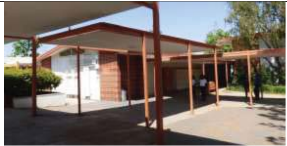
Building 17, South and West Elevation, View Northeast
