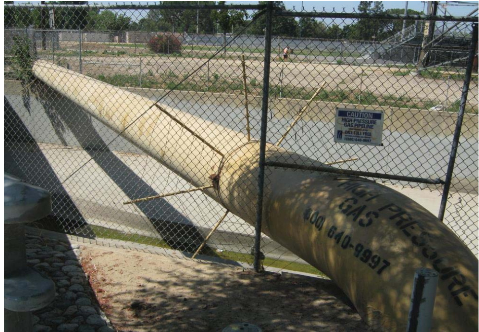
Photograph 23: View of high pressure natural gas pipeline over the Aliso Canyon Wash, adjacent to the east of the site.
