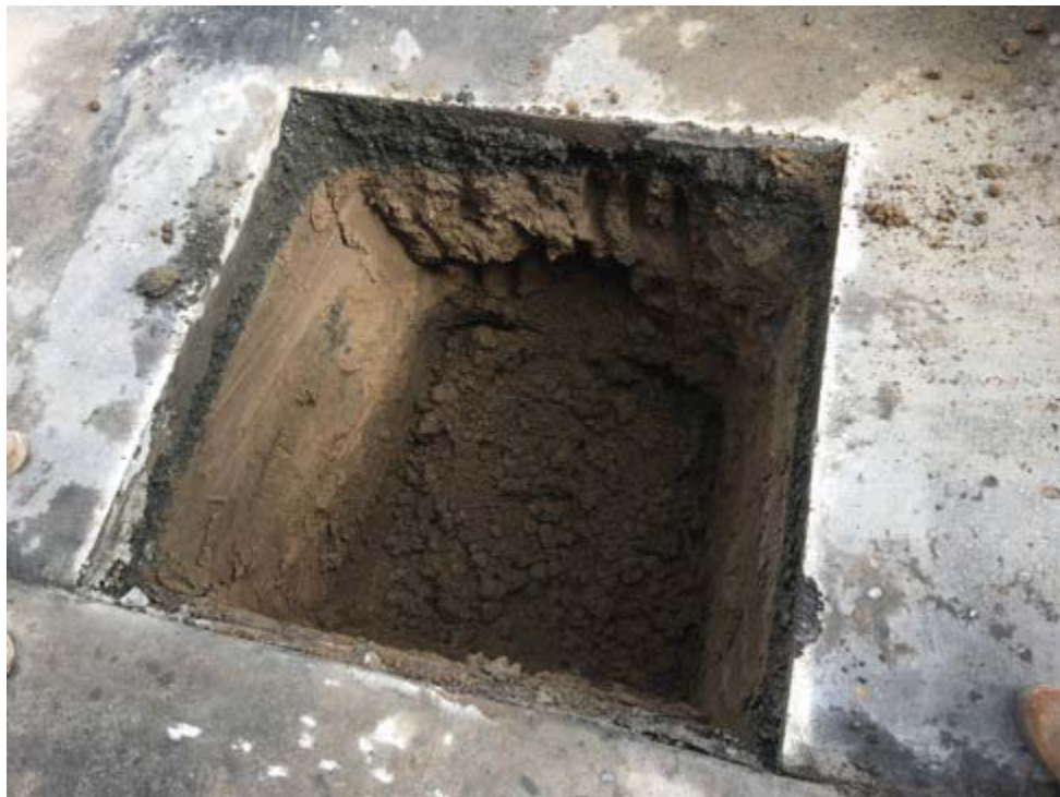
Photograph 6 – Vapor probe SV2 after excavation.
