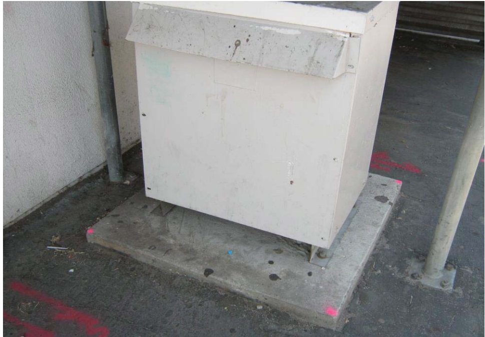
Photograph 17: View of typical small pad-mounted transformer at the site.
