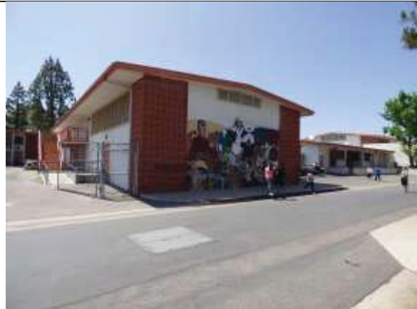
Classroom Building 18, East and South Elevation, View West
