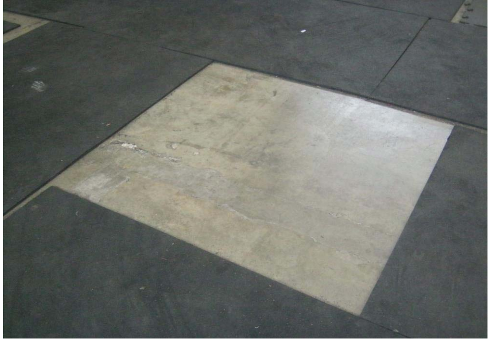
Photograph 13: View of suspected former hydraulic lift in Room N2 of Building N.
