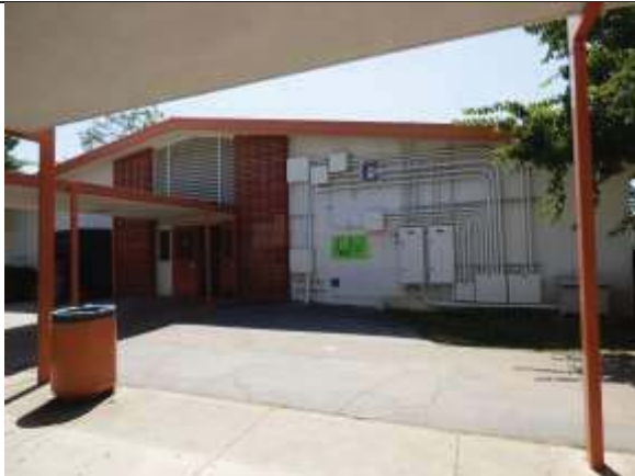
Administrative Building 6, East Elevation, View West
