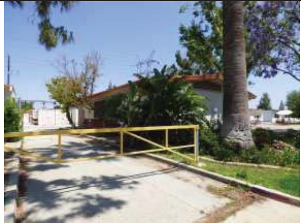
Building 13, West and North Elevations, View East
