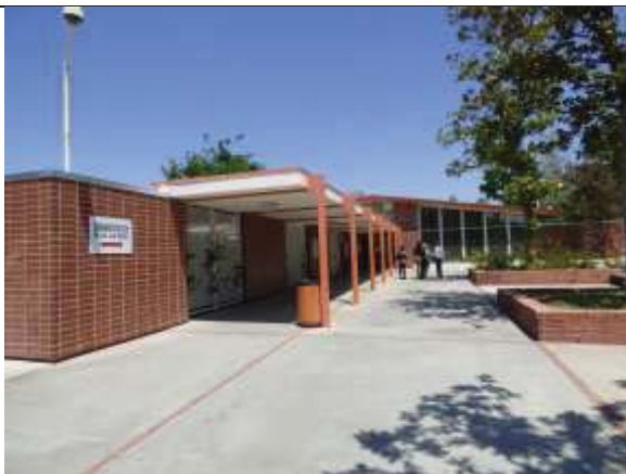
Administrative Building 6, Primary (West) Elevation, View East
