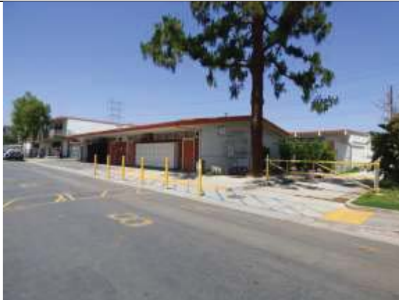
Building 11, West and South Elevations, View East
