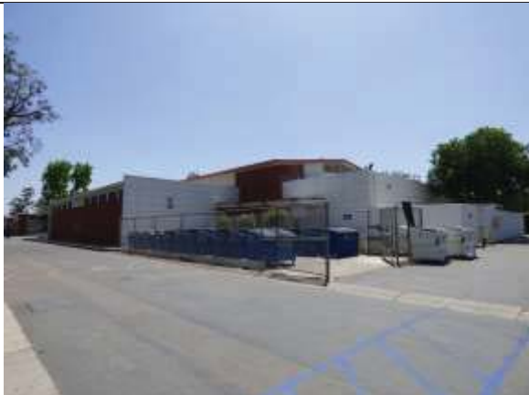
Multi-Purpose Building 14, North and East Elevation, View Southwest
