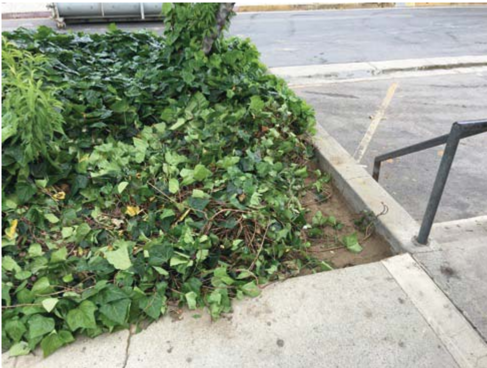
Photograph 2 – Boring B7 location after backfilling.
