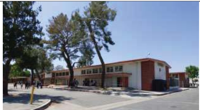
Classroom Building 20, East and South Elevation, View Northwest
