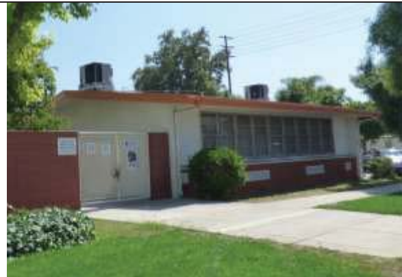
Classroom Building 1, North and East Elevation, View Southwest
