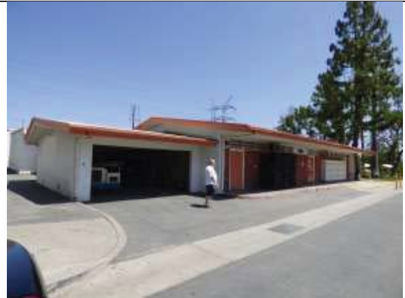
Building 11, West and North Elevations, View East
