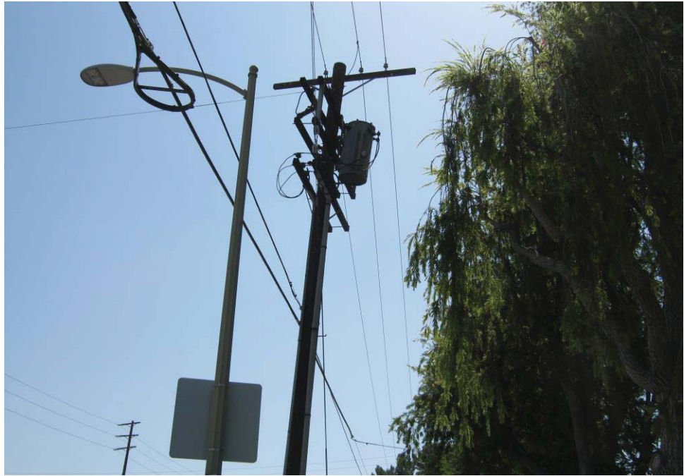
Photograph 19: View of pole-mounted transformer along Roscoe Boulevard, north of the site.
