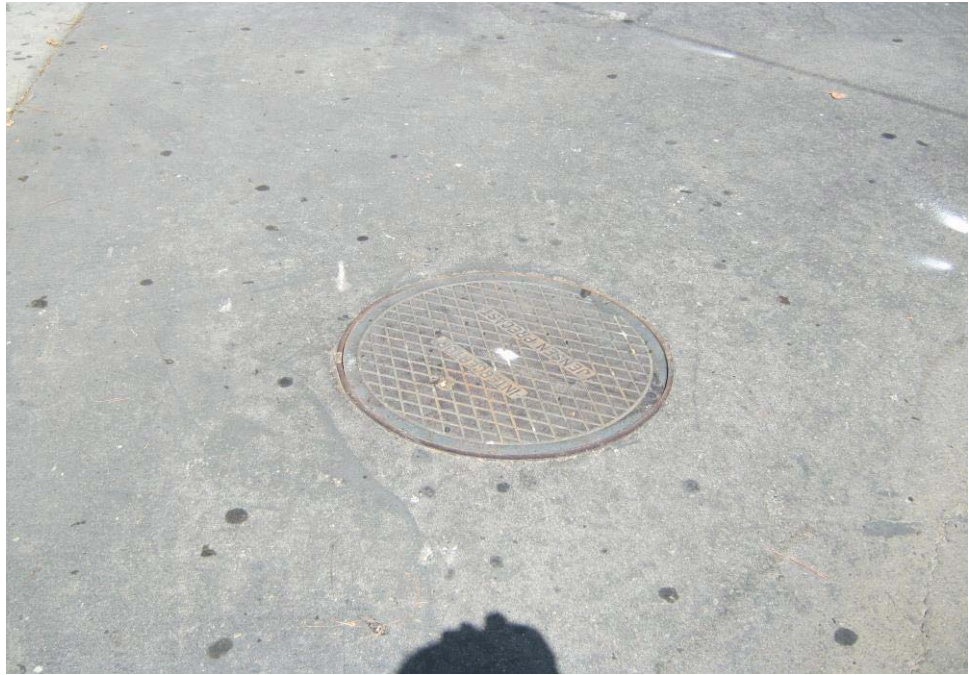
Photograph 15: View of interceptor north of Media Center Building.
