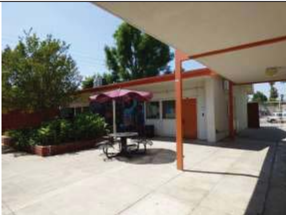
Classroom Building 1, South Elevation of Building 1, View North
