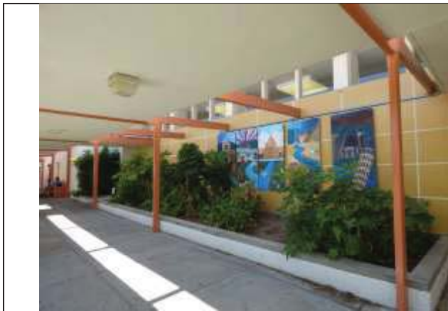
Library Building 2, East Elevation, View West
