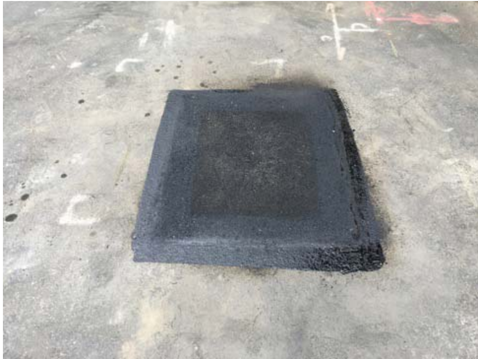
Photograph 5 – Boring B54 after backfilling and paving.
