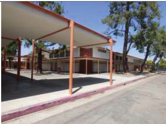
Classroom Building 20, West and South Elevation, View Northeast
