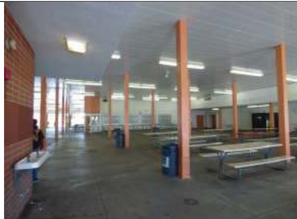
Multi-Purpose Building 14, Underneath Canopy, View Northeast
