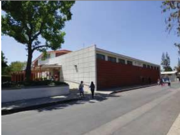
Multi-Purpose Building 14, South and East Elevation, View Northwest
