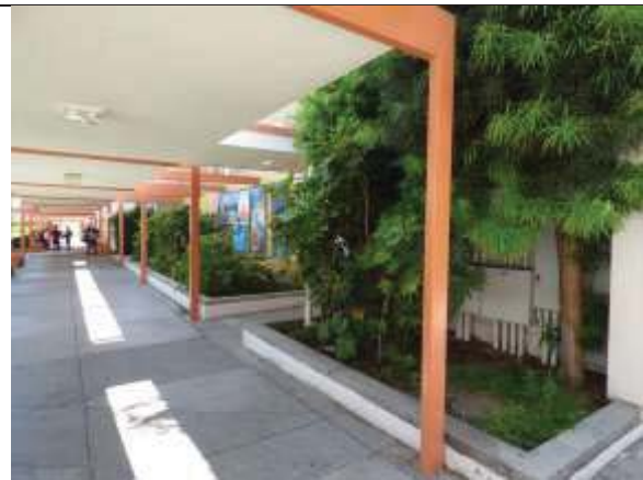
Library Building 2, East Elevation, View Southwest
