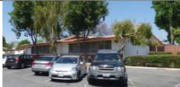
Classroom Building 3, West Elevation, View East
