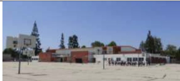
Physical Education Building 21, Rear (South) Elevation, View Northwest
