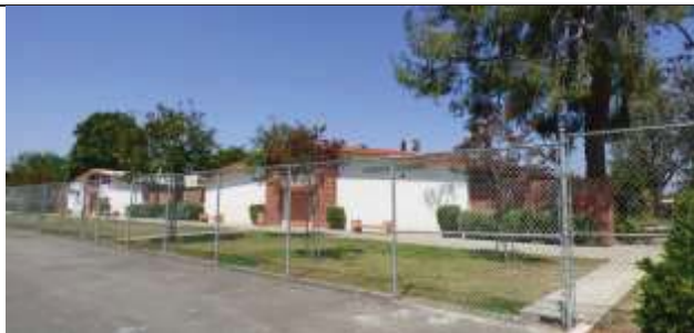
Buildings 4 to 5, View Northeast
