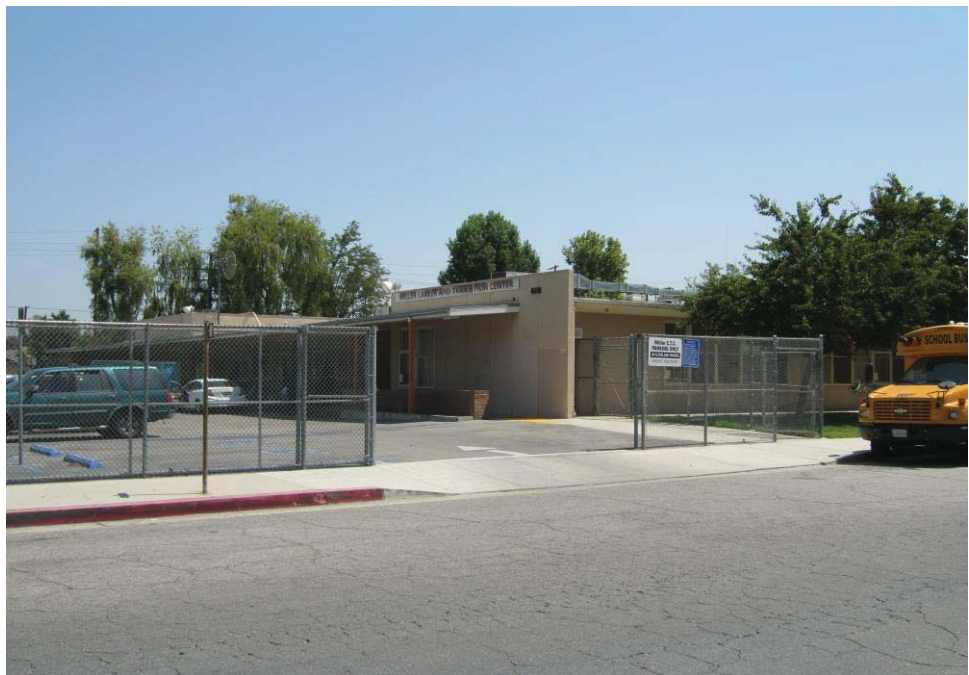
Photograph 2: Looking north at the Miller Career and Transition Center in the northern portion of the site.
