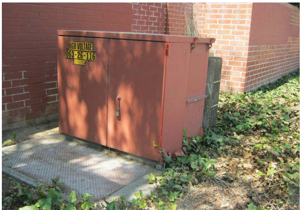
Photograph 18: View of large pad-mounted transformer adjacent to the north of the Miller Career and Transition Center.
