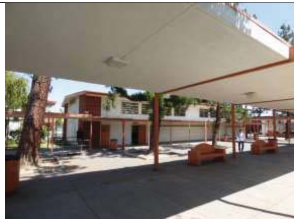
Classroom Building 20, North and West Elevations, View East
