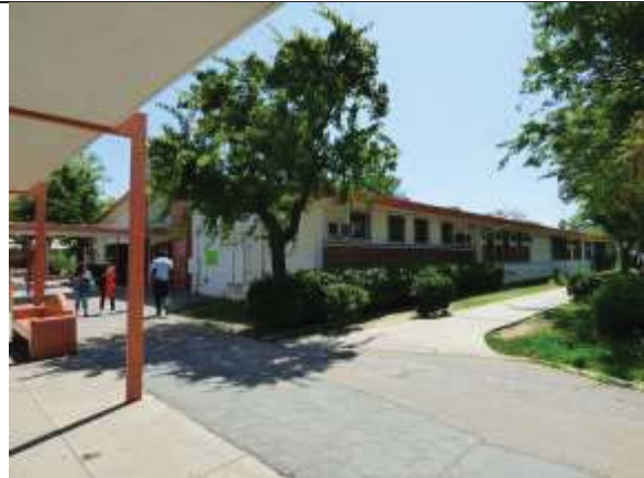
Administrative Building 6, North Elevation, View Southwest
