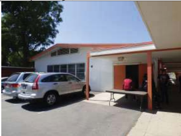
Library Building 2, South Elevation, View North
