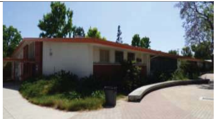
Classroom Building 3, North Elevation, View Southwest
