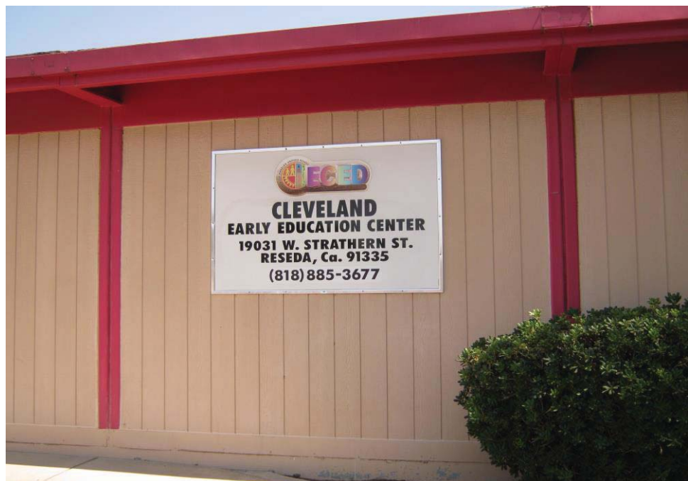
Photograph 4: View of Cleveland Early Education Center in the southern portion of the site.
