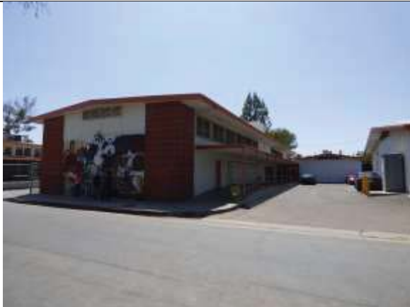
Classroom Building 18, East and North Elevation, View West
