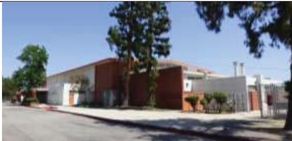
Physical Education Building 21, North Elevation, View Southwest
