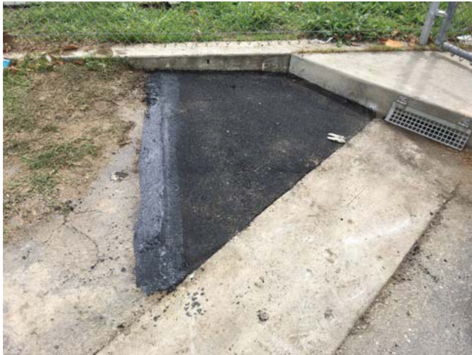
Photograph 10 – Boring B58 after backfilling and paving.
