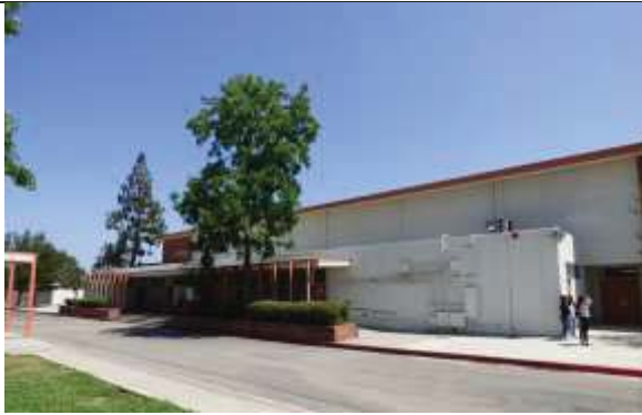
Physical Education Building 21, Primary (North) Elevation, View Southeast
